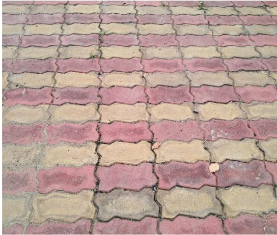
Paving stone installed in campus
