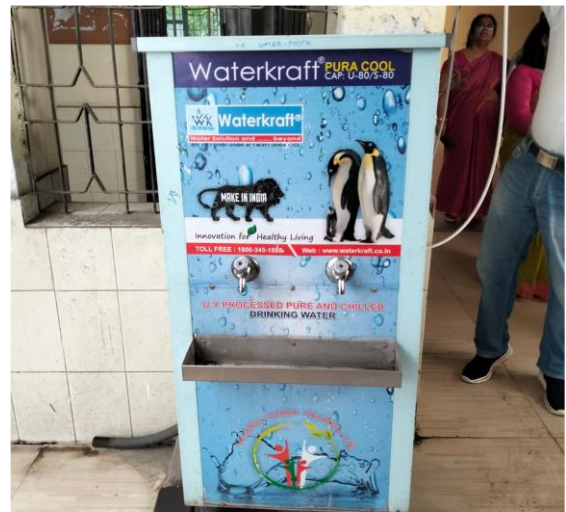
Push taps installed
