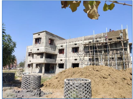
Under Construction Hostel For the Students of Minority Community
