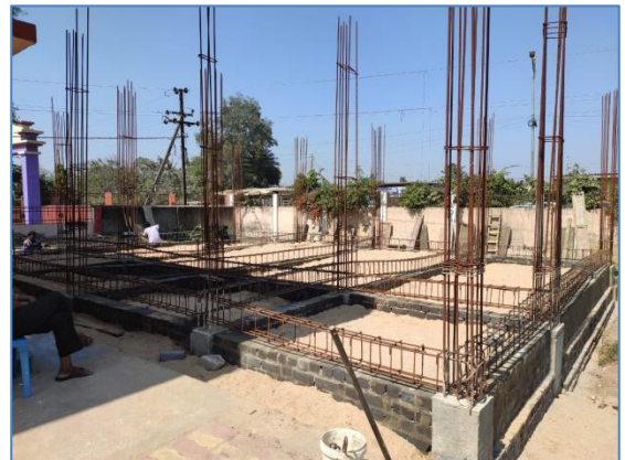
Under Construction Building For Bank-2
