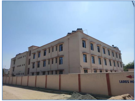
Newly Constructed Girl's Hostel No-3
