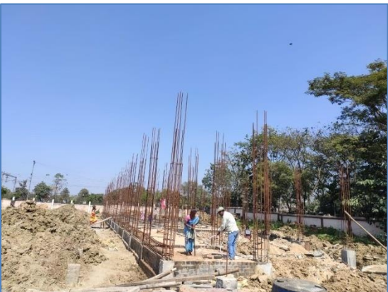
Self-Financing Block Under Construction -1
