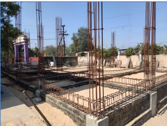
Under Construction Building For Bank-1
