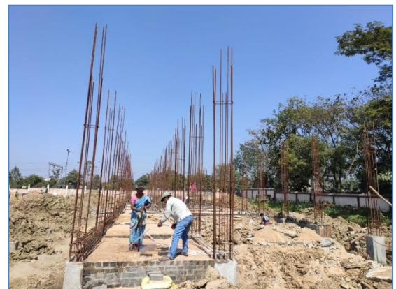
Self-Financing Block Under Construction -2
